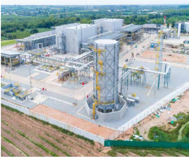
Project Name: PTT Midline Compressor Station
