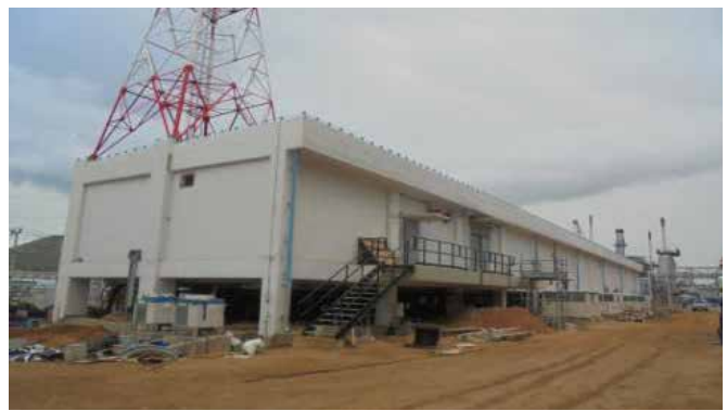
Project Name: Thai Oil LAB
