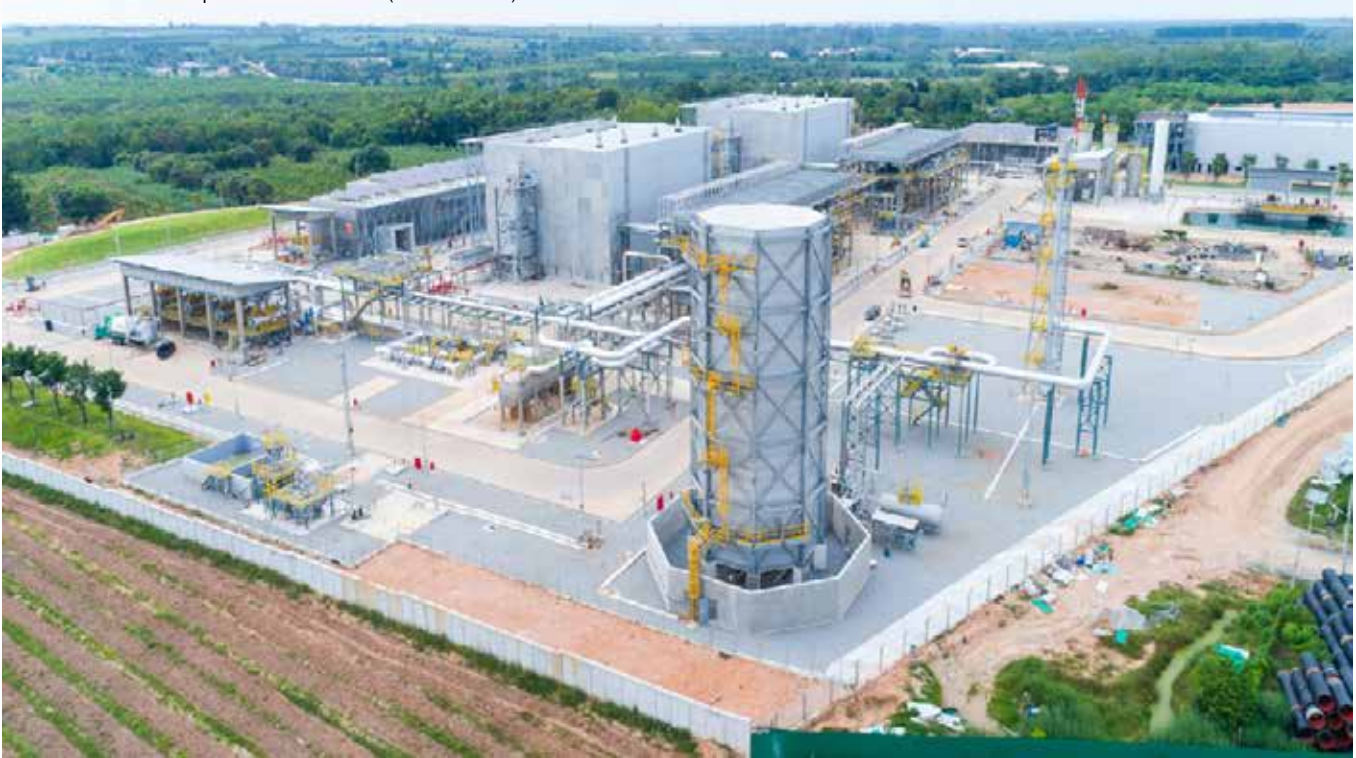
PTT Midline Compressor Station (SMP / E&I)
