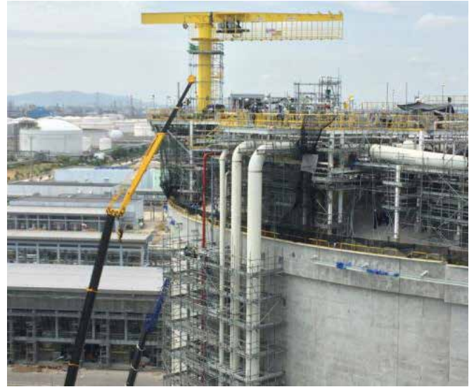
Project Name: PTT LNG Receiving Terminal Expansion
