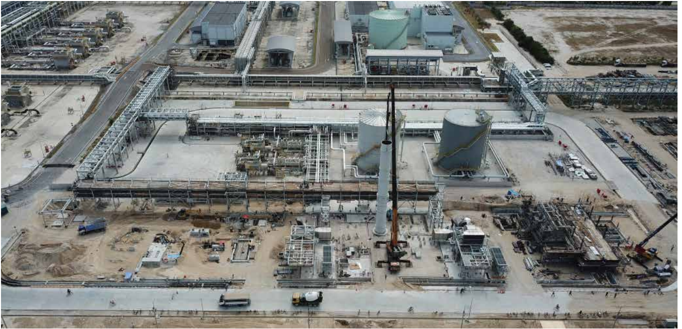
Project Name: PTT LNG Cold Water Facilities
