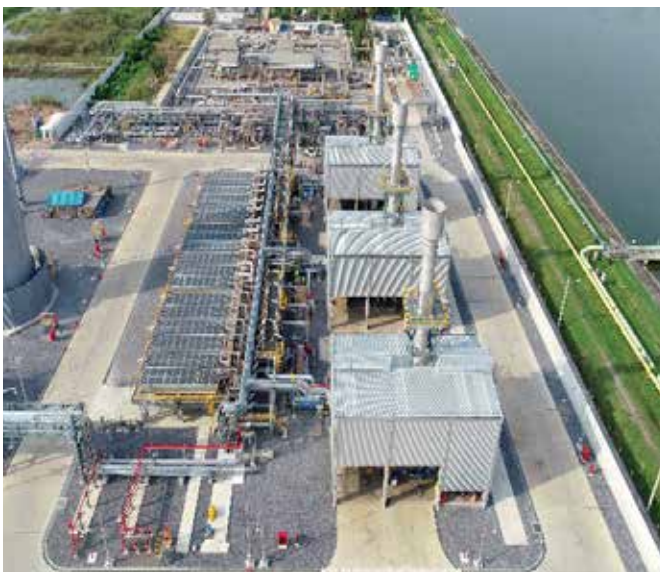
Project Name: PTT Wangnoi Compressor Station
