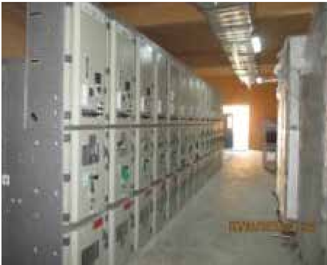
Project Name: PTT LPG Terminal Khao Bo Ya E&I
