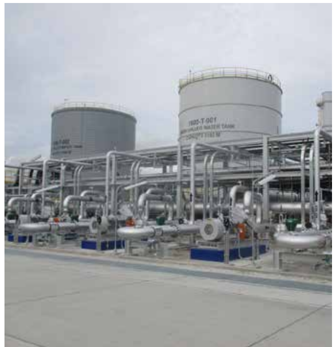
PTTLNG Cold Water Generation Plant (EPC)
