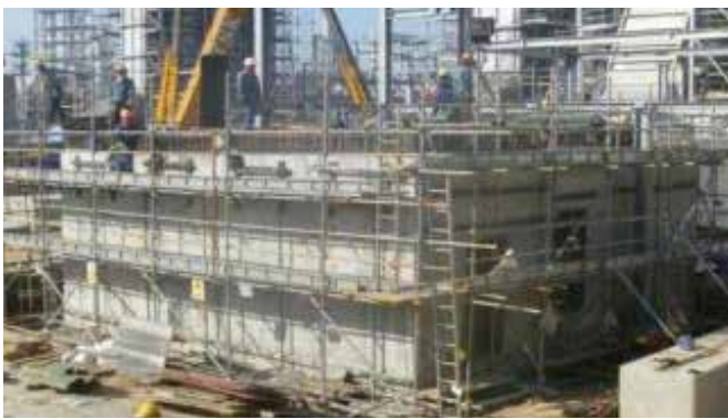
Project Name: TOP 202MW Small Power Producer Building
