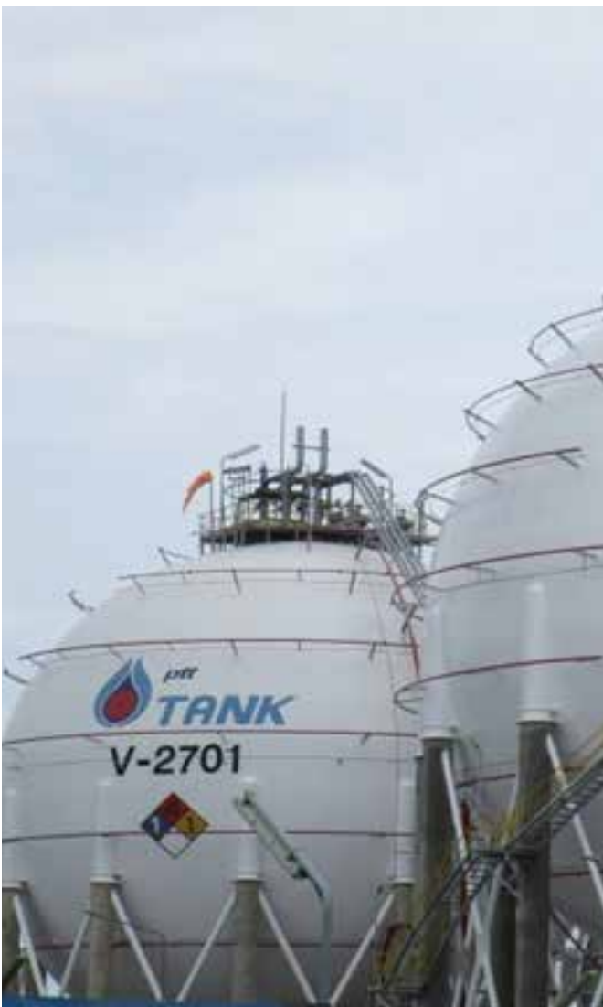
Project Name: PTT Tank Terminal
