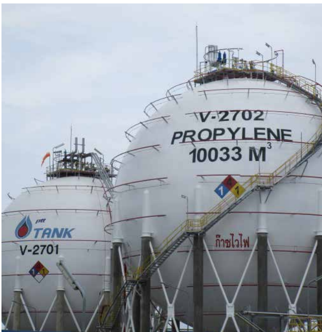
PTT Tank New Propylene Storage Tank(EPC)
