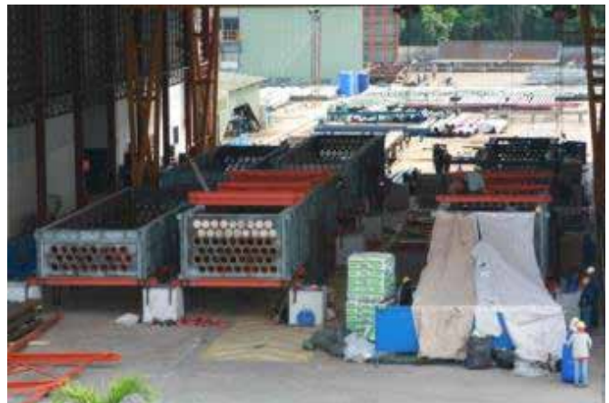
Heat Exchanger Fabrication
