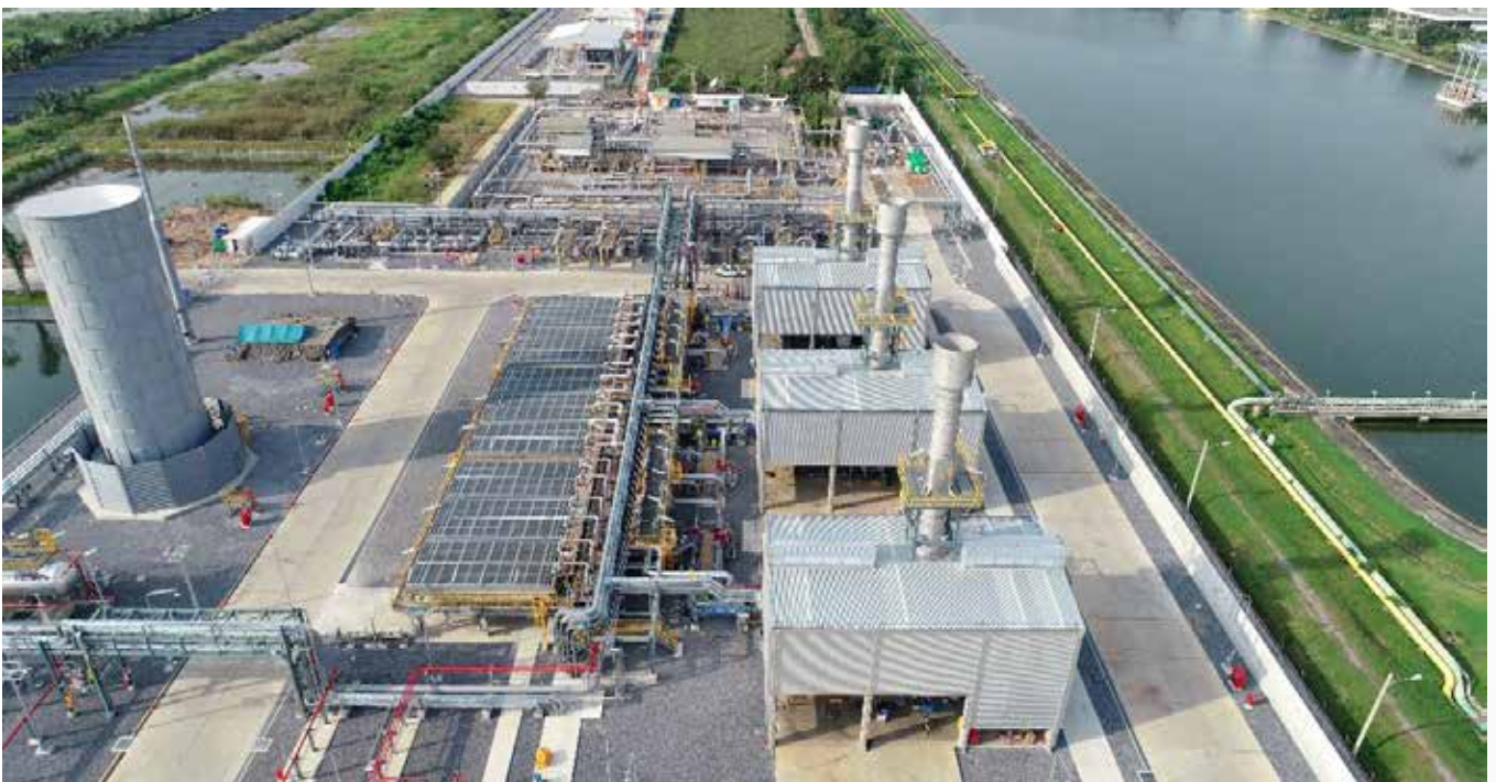
PTT Wangnoi Compressor Station (Civil & SMP)
